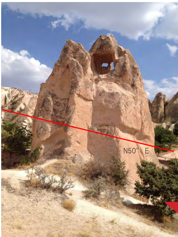
Figure 7. the rock surface caused by fault (north side of church)
