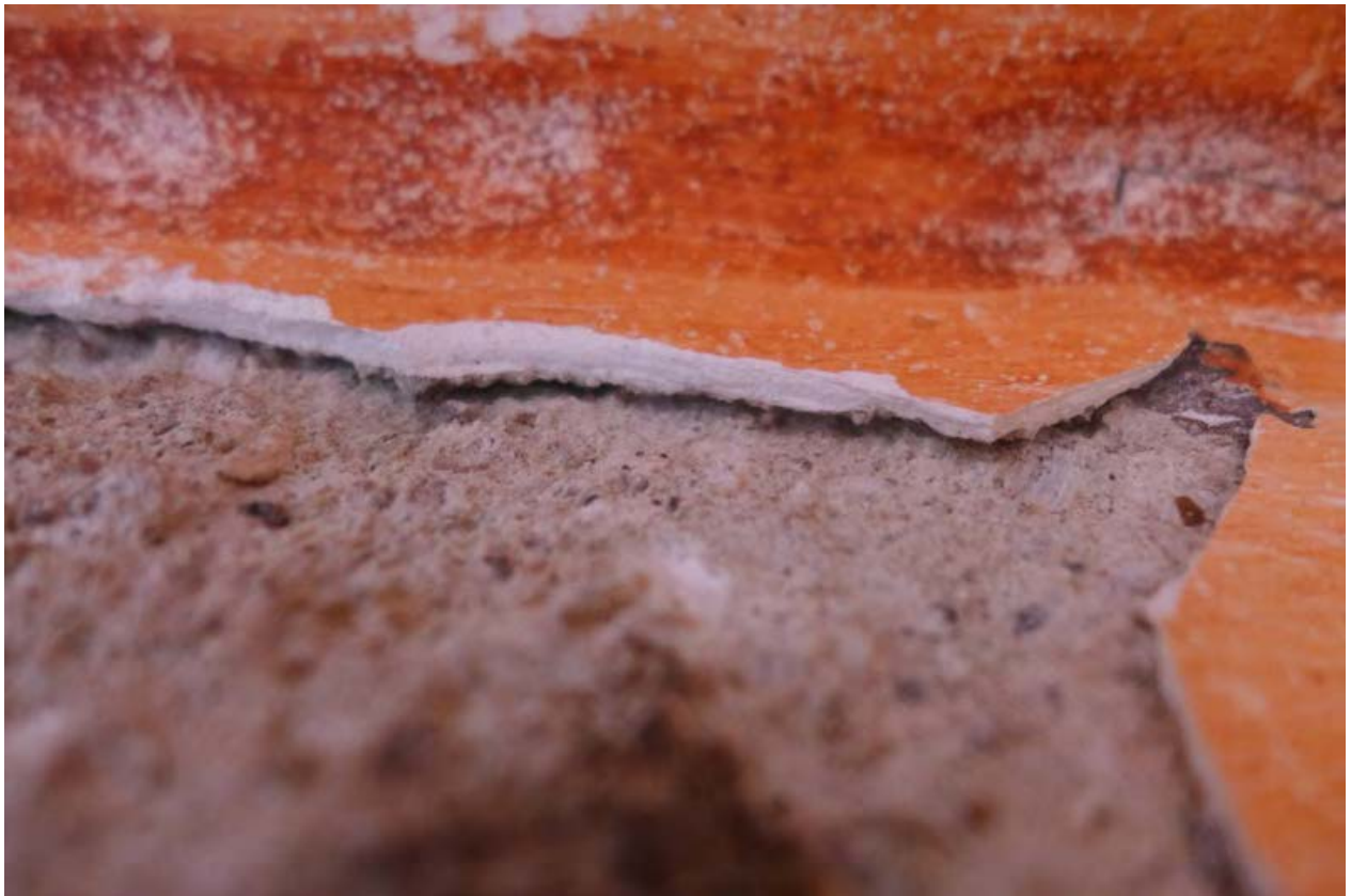
Figure 17. Area of delamination associated with mechanical damage
