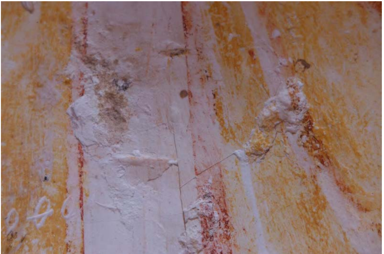
Figure 25. The painting stratigraphy has remained intact despite impact damage
