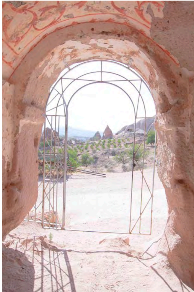
Figure 13. Metal door which secures the entrance to the church
